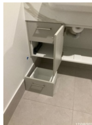
#575 | Level 03 > 50 > Bathroom | Cabinet Maker Fit bottom drawer in track
