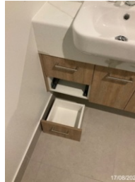
#606 | Level 03 > 49 > Bathroom | Cabinet Maker Fit bottom vanity drawer in track
