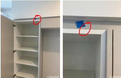
#599 | Level 03 > 49 > Kitchen | Cabinet Maker Touch up chip on filler panel above pantry
