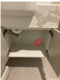
#574 | Level 03 > 50 > Bathroom | Cabinet Maker Fit screw cover in vanity cabinet
